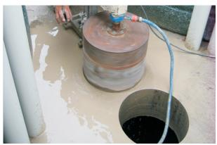
Bit sizes: 2", 2.5", 4.25", 5", 6", 7", 8", 12" & 16" Coring depth up to 10" for most sizes
